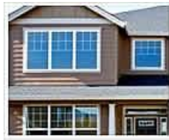
Building envelope, residential new construction and retrofits
